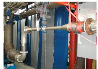
Level 6: If straight pipe run is very short and/or if pipe diameter is big and/or if requirements on accuracy are high, a multiple sensor calibration is used to improve accuracy of flow reading. Calibration is customized and considers all conditions at site.
