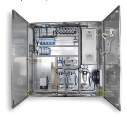
The gas composition in agricultural biogas plants varies depending on the process and composition of feedstock. Biogas quantity and quality are measured after the individual fermenters, at the flare, are used for filter monitoring in gas purification and before consumers such as boiler and CHP. Another application is monitoring the quality of the supplementary air from the double membranes of the fermenter covers.
